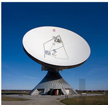
Fig.2: Parabolic Reflector Antenna
